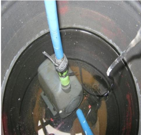
**Gambar 6. Pompa Air**
